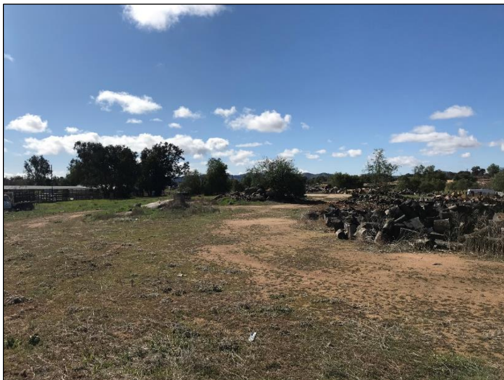
. Figure 13. Project overview from northern boundary, view south
