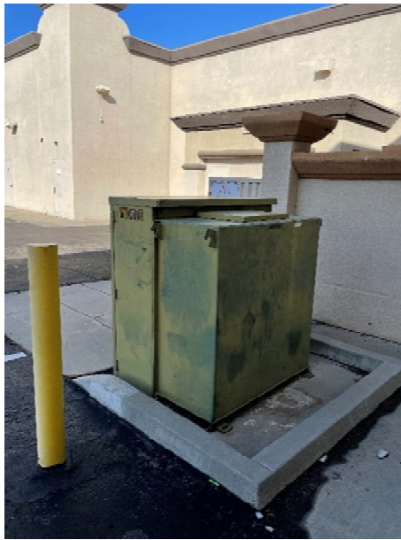
Left: Transformer located in the parking lot at the northwest corner of the Site | Middle: Transformer located at the southwest building exterior | Right: Label indicating that transformers were “filled with non-PCB dielectric fluid at time of manufacture” observed on both the above transformers.
