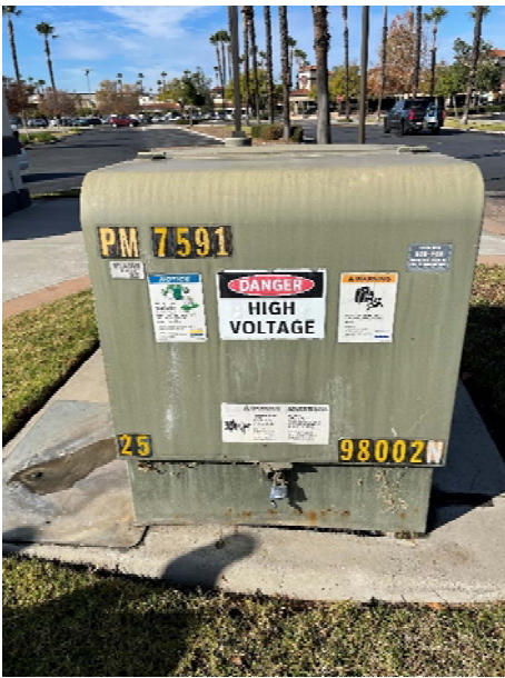
Left: Transformer located in the parking lot at the northwest corner of the Site | Middle: Transformer located at the southwest building exterior | Right: Label indicating that transformers were “filled with non-PCB dielectric fluid at time of manufacture” observed on both the above transformers.
