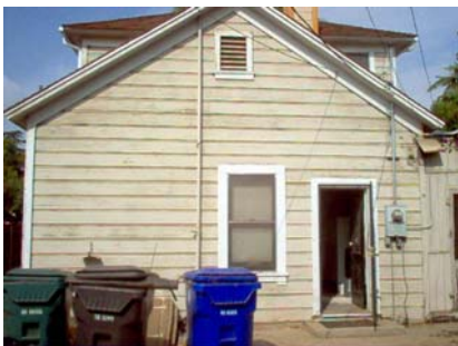
West Elevation View West
