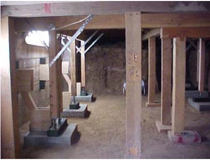
Shoring the Basement
