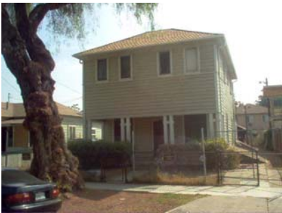
West Elevation View East
