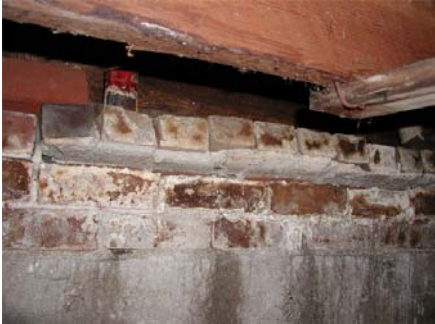
Brick and Concrete Wall in Basement
