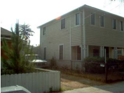
North and West Elevation View Southeast
