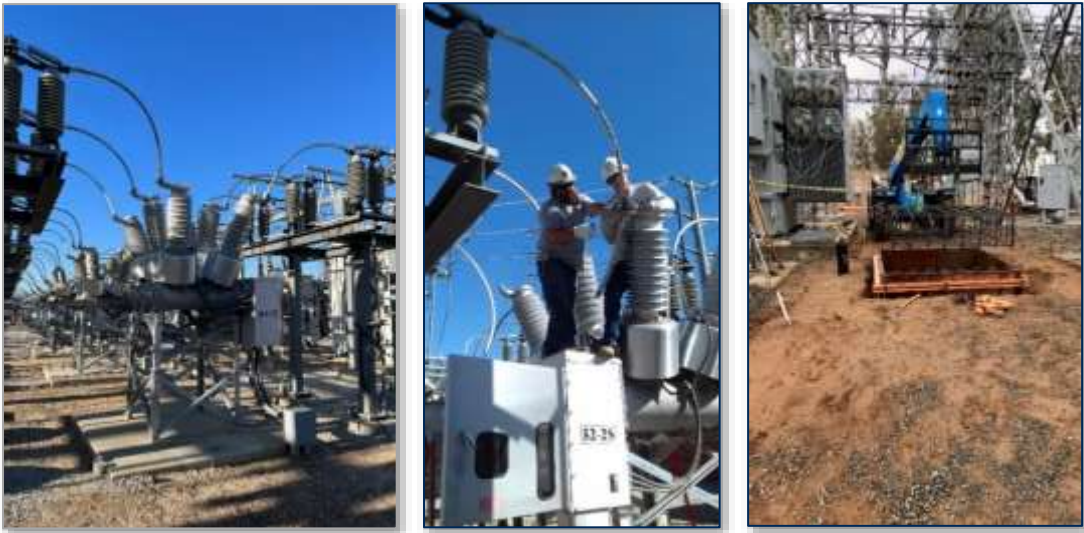
Breaker Replacement at Substations
