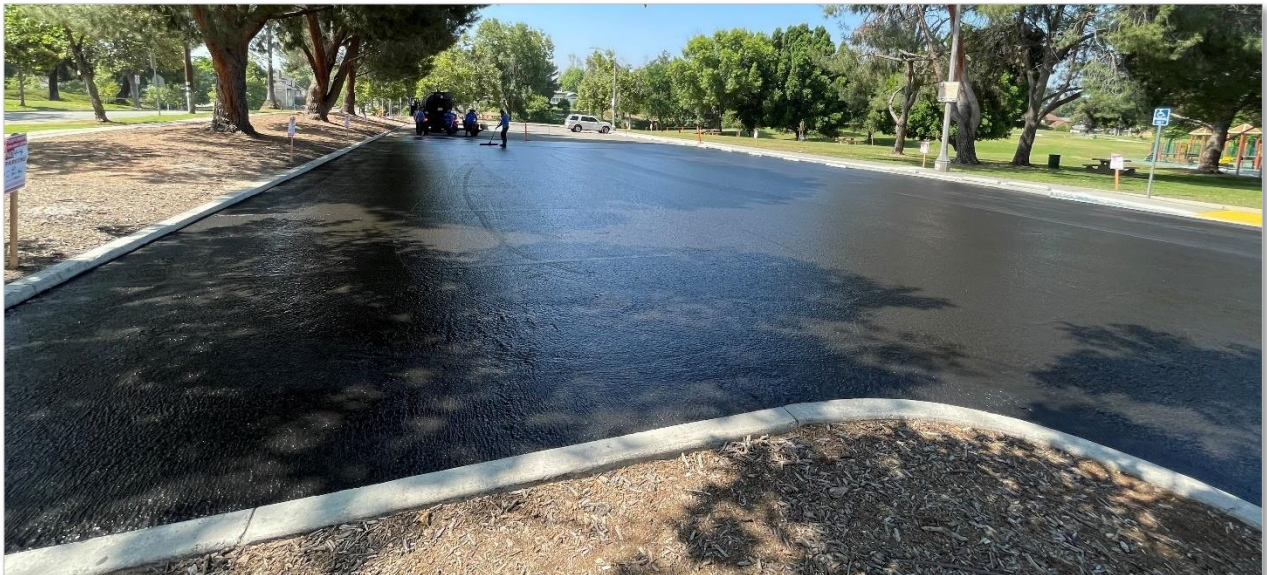
Bordwell Park Slurry/Stripe Parking Lots
